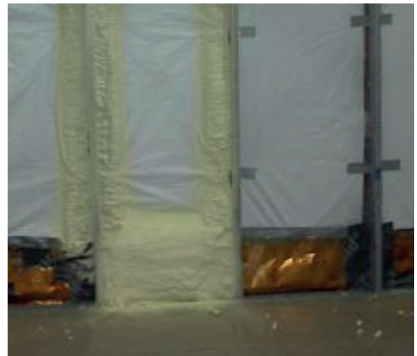
FIGURE 6. Use of a membrane material to create a drainage plane.
